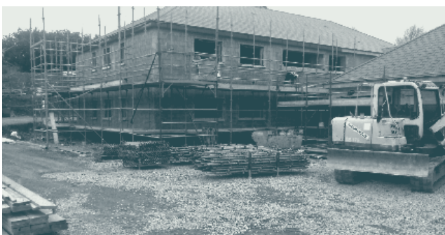
Fellowship House, six months into build
