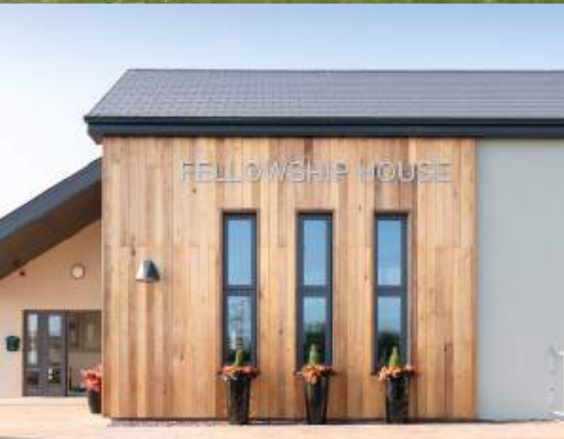
TABOR FELLOWSHIP Secondary Residential Treatment Centre
